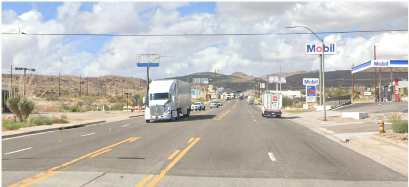
Figure 2-11: West Beale Street Existing Cross-Sectional View, Source: Google
